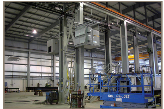
SmogHog systems are arranged in a racetrack configuration.
